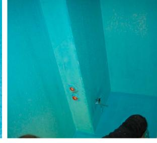
When starting a waterproofing job, one must follow the national building regulations as well as the instructions given by the waterproofing membrane manufacturer. It is crucial to ensure sufficient membrane coverage and layer thickness over the surfaces. When calculating the membrane coverage, one must take into account substrate's porosity and reinforcing fabrics used.
