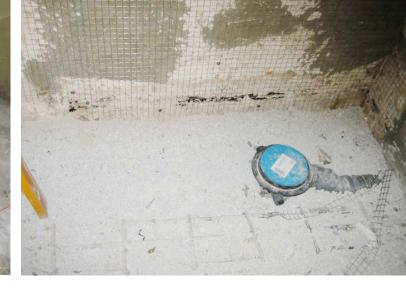
When renovating a block of flat, one has to consider the entire floor construction. Do we need to remove and replace the filling materials? Is the construction strong enough to bear the new floor construction? How to install new drain and water pipes?
