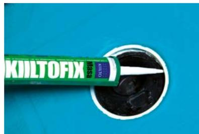
**11.** Seal the junction between the tension ring and floor drain with Kiiltofix Masa. Kiilto Kaivolaippa's compatibility with most floor drain types is tested and approved.
