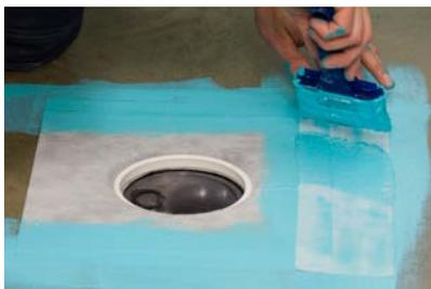
**9.** Kiilto Kaivolaippa has reinforcements on two sides, apply Kiilto Kerafiber on them. Another two sides must be reinforced with reinforcement tape. See that the tape overlaps Kaivolaippa for minimum 30 mm.
