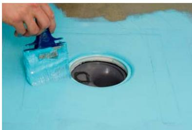
**10.** Apply Kiilto Kerafiber over the entire floor area and around the tension ring.
