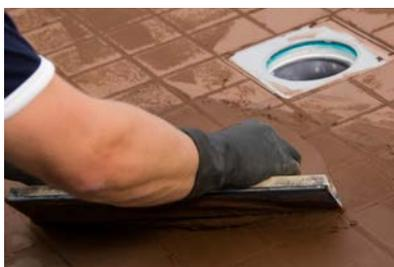
**13.** Apply Kiilto Saumalaasti with a rubber trowel and press it in the joints. Wait for 15-30 minutes and wash away excess grout with a damp sponge. Use a damp sponge, since too much water can discolour the joints. Wall joints' profile can be finished using a thick electric wire.
