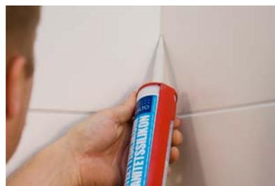
**14.** Wipe away any excess grout from corners and seam them as well as pipeline inlets with Kiilto Saniteettisilikoni. Let cure until the next day before using the new bathroom. Keep the underfloor heating system turned off approx. 7 days. Bring the system up to its operation temperature gradually in stages over a few days.
