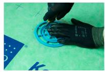
**4.** Wait at least 2 hours after the foil installation before cutting a hole for the floor drain and starting tiling.
