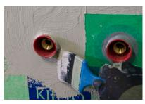
**5.** Inlets need not to be measured accurately, since they will be covered with a prefabricated reinforcement piece with KeraSafe Speed A+X adhesive.
