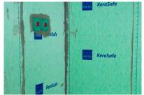
**7.** As the last foil is installed, you can start tiling. Start the tiling from the same wall as you started laying the KeraSafe + foils.
