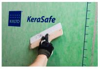
**4.** Press the foil tightly onto the substrate and rub into position with a rigid plastic trowel so that all air is pressed out and the foil is 100 % adhered to the substrate.
