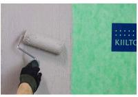
**2.** Lay Kiilto KeraSafe + foils one by one with Kiilto KeraSafe Speed A+X adhesive.
