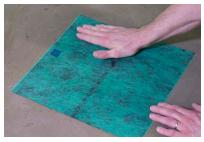
1. Install Kiilto KeraSafe Kaivolaippa reinforcement on the floor drain before laying KeraSafe + foils.
