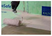
**2.** Start laying KeraSafe + foils on the floor in the same manner as on the walls: one by one with min. 5 cm overlaps.
