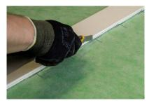
**1.** Before you start, cut the required number of KerSafe + foils ready for the job. If you need more open time for the foil installation, prime the substrate. Mix liquid A and powder X components of the adhesive carefully. The pot life of a mixed product is min. 1 h and coverage approx. 12 m².
