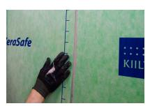
**3.** Lay every foil at least 5 cm over the previous one. The lower edge of the foils must stretch 5 cm on the floor.
