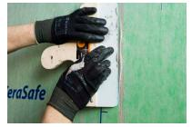
**6.** Lay the next foil and carefully rub onto the substrate. The adhesive oozing out of the seams can be levelled out on the foil surface.
