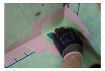
**3.** Corner reinforcements are fixed with KeraSafe Speed A+X adhesive.
